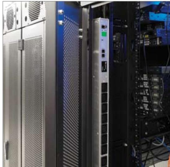
**Figure 4. Racks with vertically mounted intelligent power strips.**
