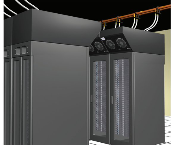
Figure 14. Supplemental cooling enables higher rack densities and improved cooling efficiency.
